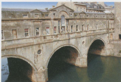
▲ Pulteney Bridge in Bath, completed in 1773. Project by Robert Adam (1728-92).
